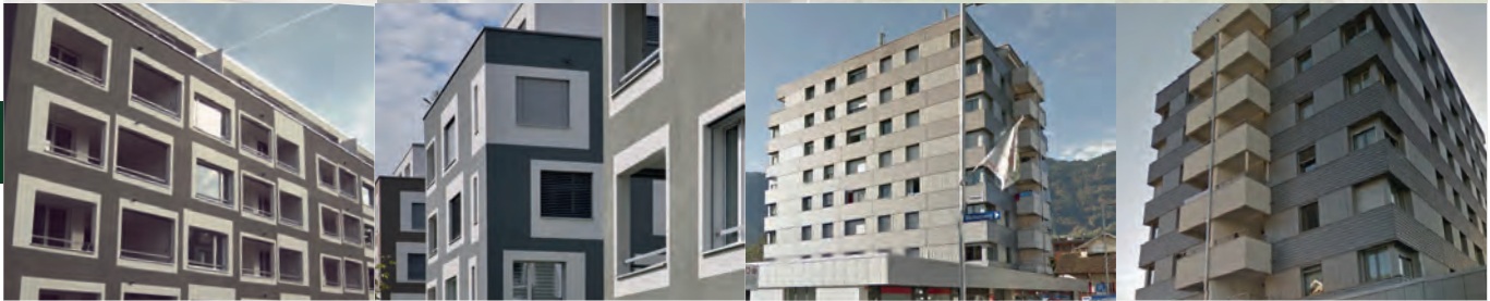
GOLDACH | SG Haini-Rennhas-Strasse 2/4/6
