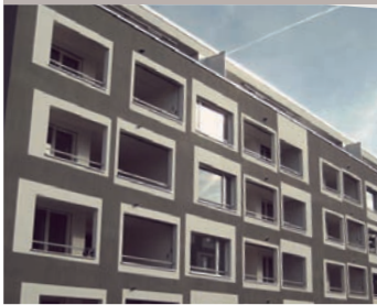
GOLDACH | SG Haini-Rennhas-Strasse 2/4/6
