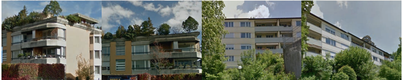
THUN | BE Neumattstrasse 21/23
