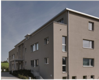
FLAWIL | SG Bogenstrasse 105/107/109
