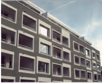
GOLDACH | SG Haini-Rennhas-Strasse 2/4/6
